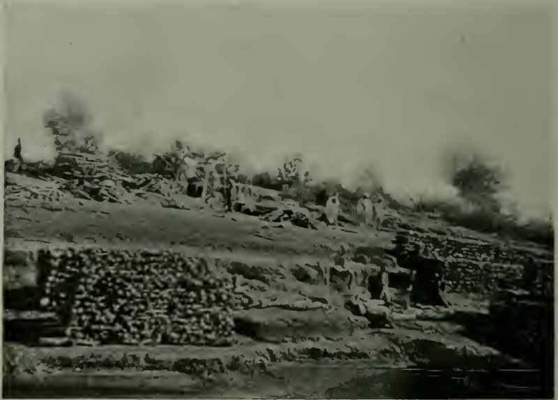
WOODING STATION ABOVE ATBARA IN 1898.
