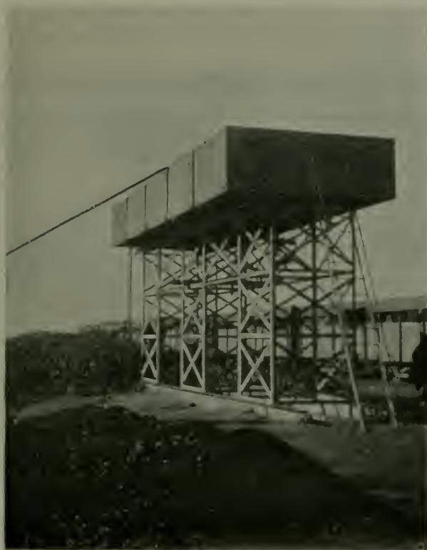
WATERING TANK AT NO. 6 STATION IN THE ABÛ-HAMED DESERT.
